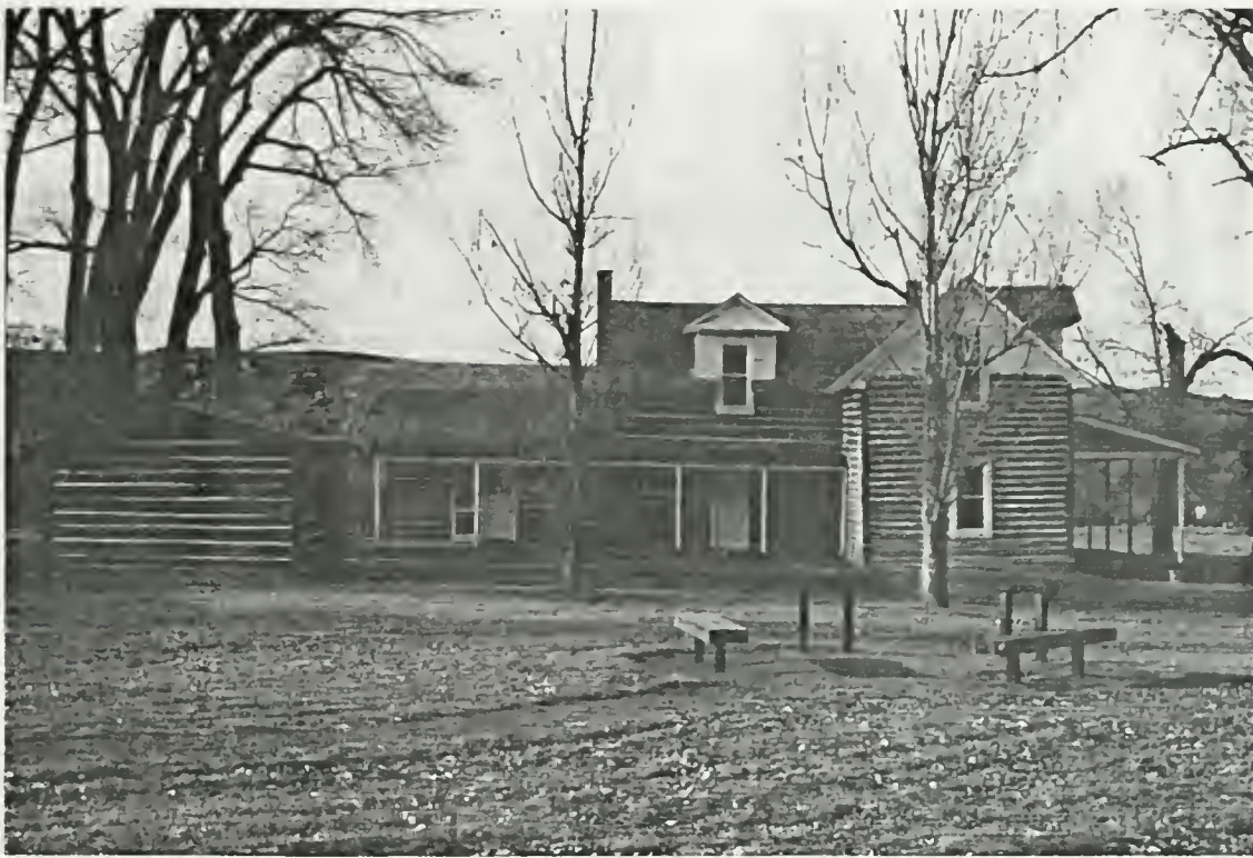
Chief's House and store after stabilization and partial restoration. Restored north porch is visible at right. Interpretive area is located in foreground.
